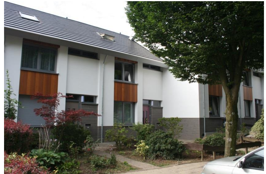
Figure: The houses after completion
