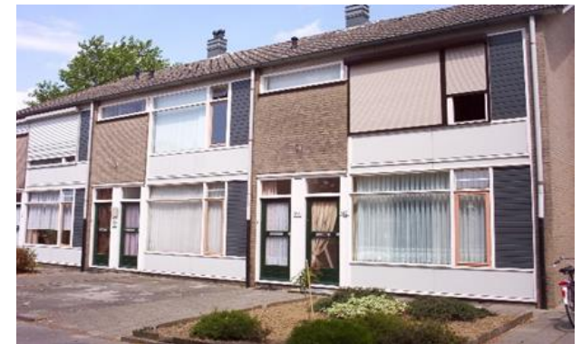
The houses before renovation
