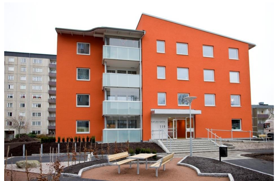
After renovation with new facade and balconies etc.
