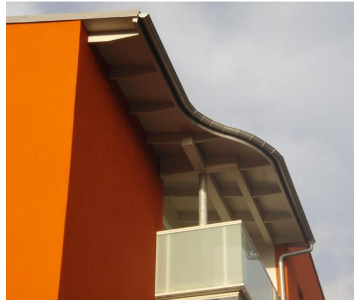
Extended eaves and balcony after renovation
