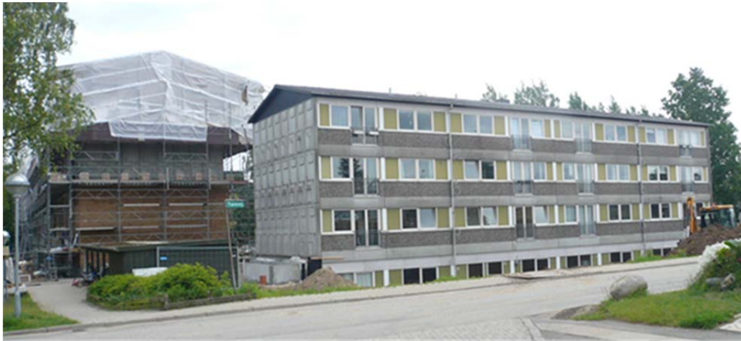
Fig. 1. Two of the three blocks at Traneparken. The photo shows the end wall of one block being renovated and the facade of the other which has not yet been renovated.
