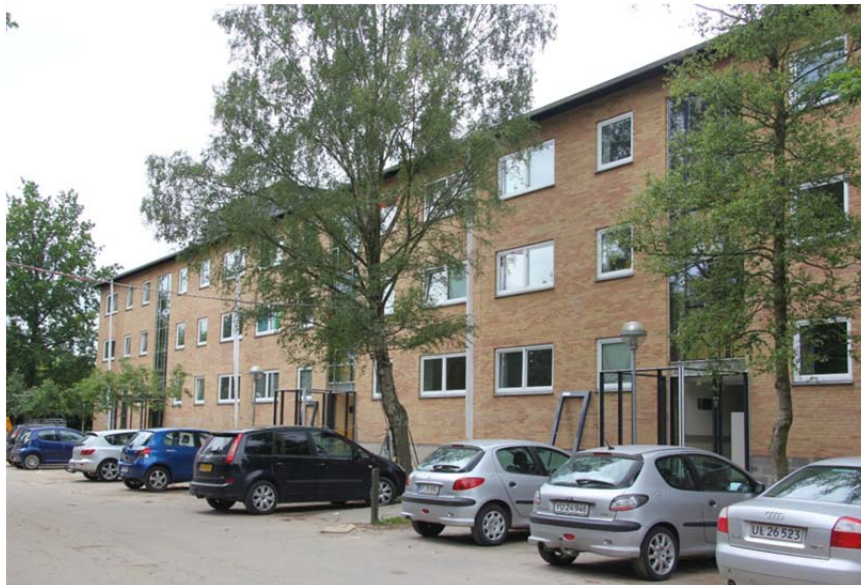
Fig. 5. Traneparken after renovation.
