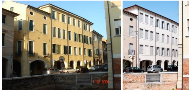
Fig. 1 General view of the building a) before and b) after the intervention.
